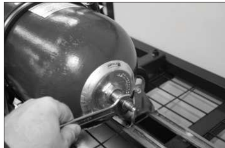
5. Remove the Gas Valve Assembly or Gas Valve Core.
